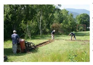
The project included installing a centrifugal pump, controller, rain sensor, three zones of drip irrigation and a yard hydrant. The water source is a nearby mountain stream.
